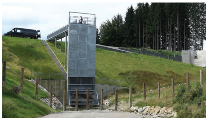
Illustration above: view into the tower construction with the vertically-operating float
