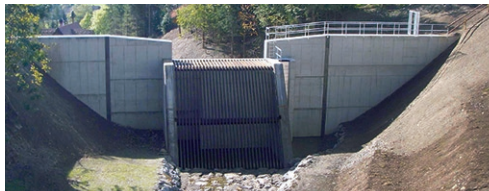
◀ Fig. 3: Rockslide break ▲ Fig. 4: Rubble catch and throttle structure ▶ Fig. 5: HydroSlide® Flow Regulator
