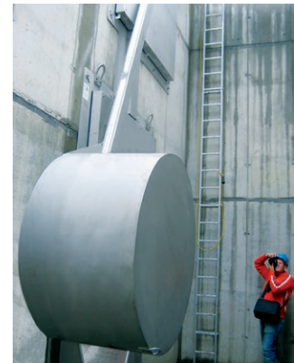
◀ Fig. 3: Rockslide break ▲ Fig. 4: Rubble catch and throttle structure ▶ Fig. 5: HydroSlide® Flow Regulator
