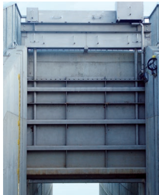
▲ Fig. 1: Fish-belly gate ◀ Fig. 2: Draining
