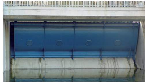
▲ Fig. 1: Fish-belly gate ◀ Fig. 2: Draining
