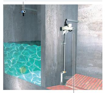
EasySlide actuator and special slide valve with connection to a central control
