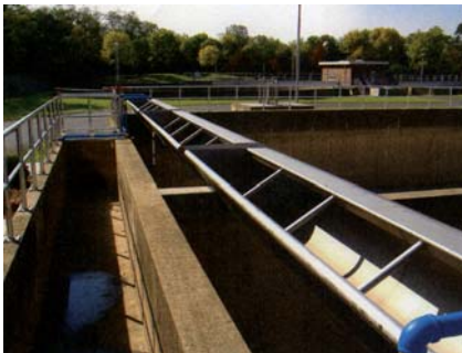
The HydroSelf tipping bucket has one or more drain holes so that stormwater cannot accumulate in open tanks.
