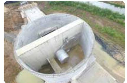
structures, or a blockage, the problem could be overcome without having to wait for the flood to subside. The ability to provide the more refined level of flow control, with relatively little maintenance, and the advantage of post-construction in-event adjustment led to the HydroSlide being adopted.
